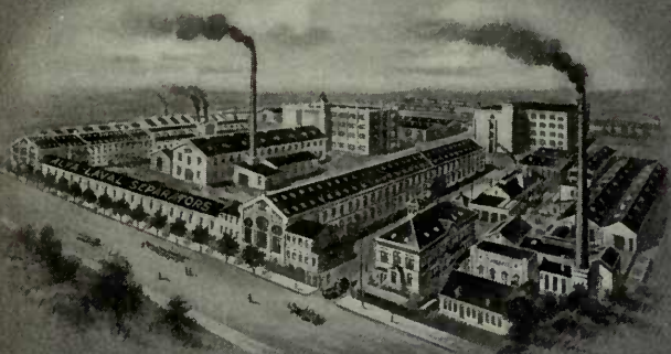
DE LAVAL SHOPS - HAMBURG, GERMANY.
